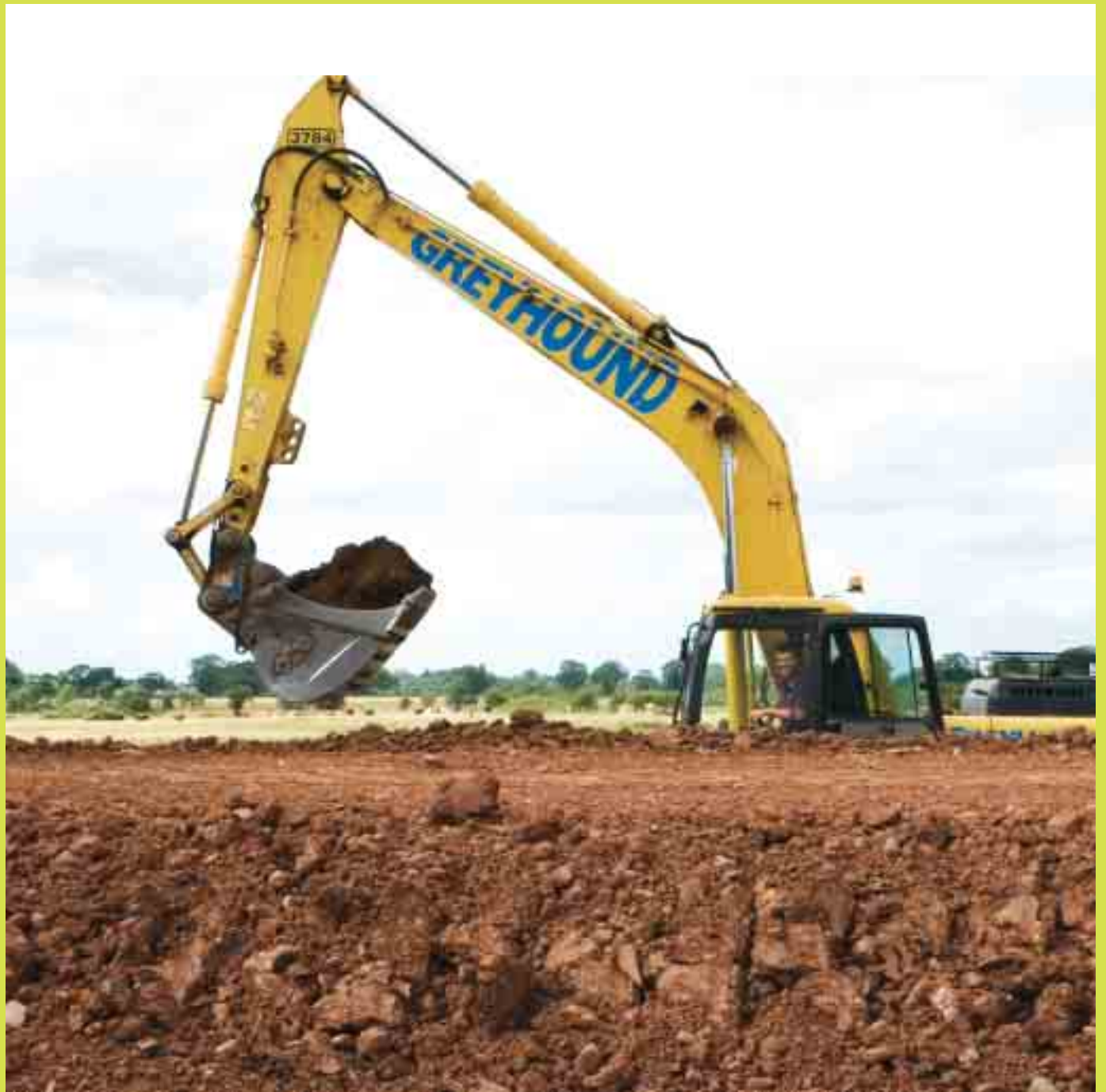
After the floods: building new £12 million flood defences in Carlisle
